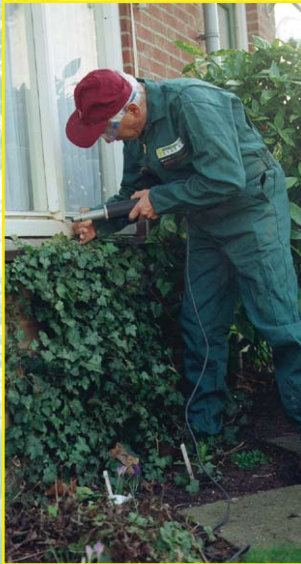
removal of excessively soft, weathered or damaged wood
