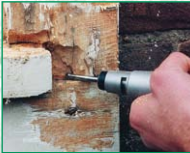
removal of excessively soft, weathered or damaged wood
